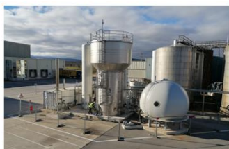
Design and construction of 110 m 3 Multi-AD 1:1 industrial-scale in a real environment
