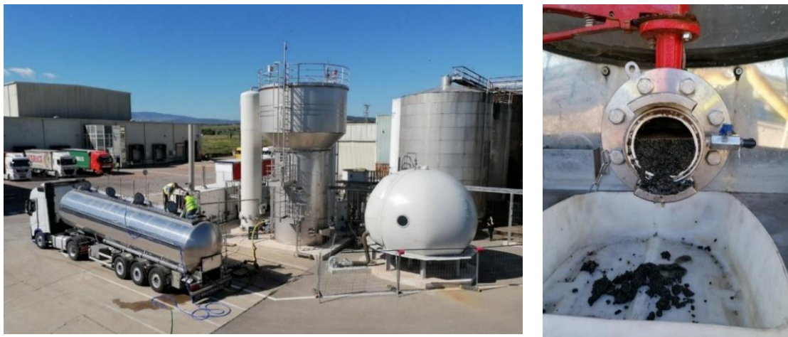
Figure 25. Images of the Multi-AD reactor seeding process.
